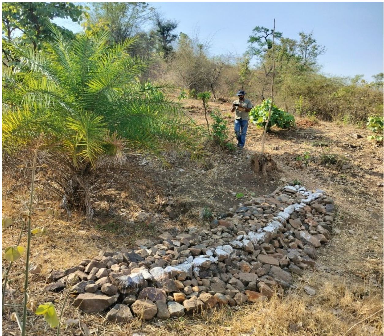
Plate 3.10: Loose Boulder Check Dam at Parasia Range of West Forest Division, Chhindwara
