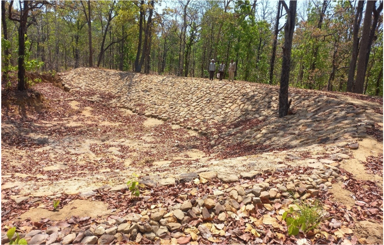
Plate 3.11: Semi Circular Percolation Tank at Delakhari Range of West Forest Division, Chhindwara
